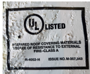
Example of Class A rating on a shingle wrapper
