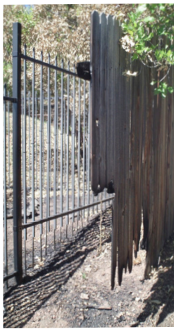
Undamaged metal fence next to a burned wooden fence
